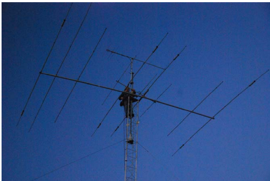
John KB0BSJ installing 2-meter and 6-meter beams Ground support provided by Marilyn Klug, Charles KI0LS, Nancy KC0YXB
